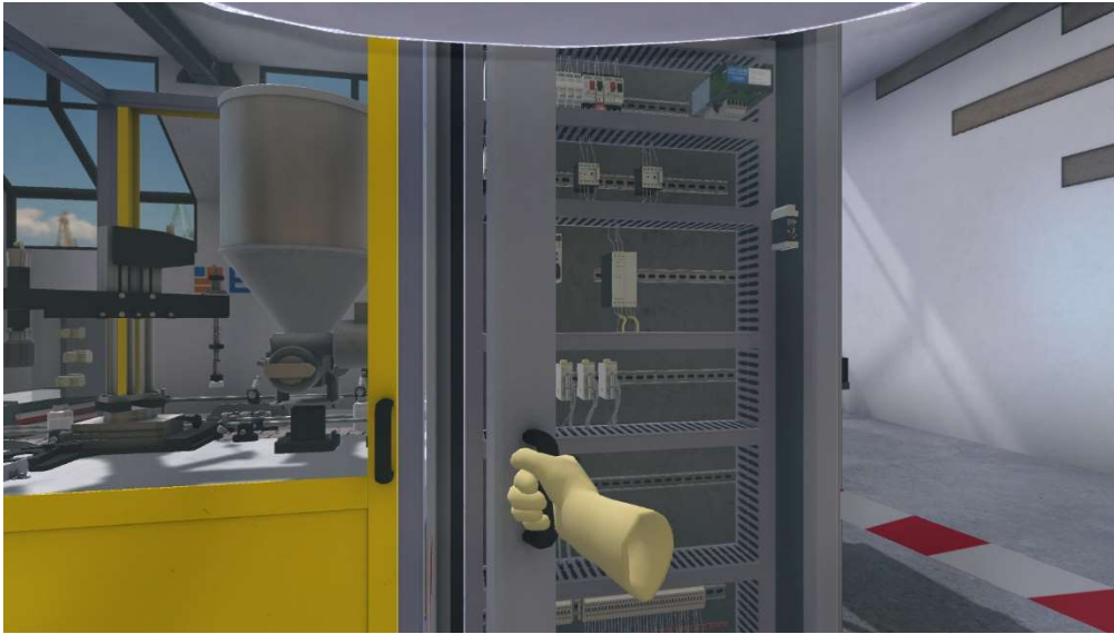
Figure 36 – Close the electrical cabinet
