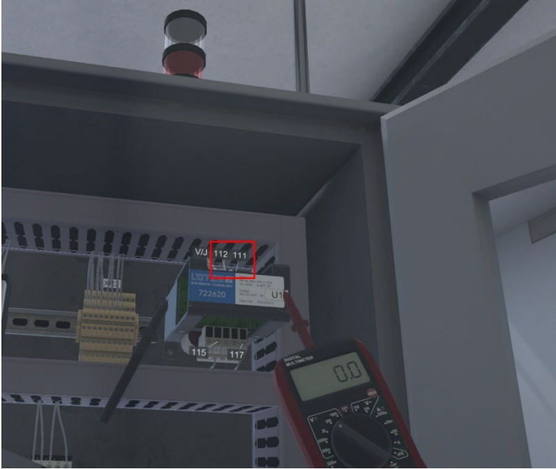
U1 Power Measurements Between Terminals 112-111
