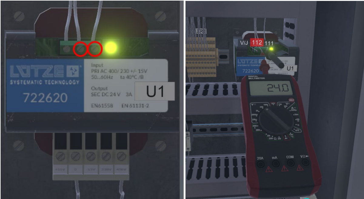
Voltage measurement at KA1 level between A1 and A2 (terminals 602 and 112 respectively)
